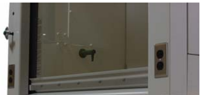
Sash with frameless PVC guides Raised airfoil; flipper style Reinforced integrated pull; raises and lowers outside the fume hood Lowers to 18"
